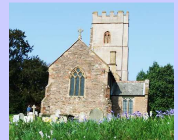
New Roof at Brompton
